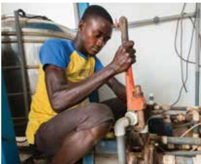
**Site operator, Humphery Aryee, repairs a leaky seal at a Safe Water Station in Pokuase.**
